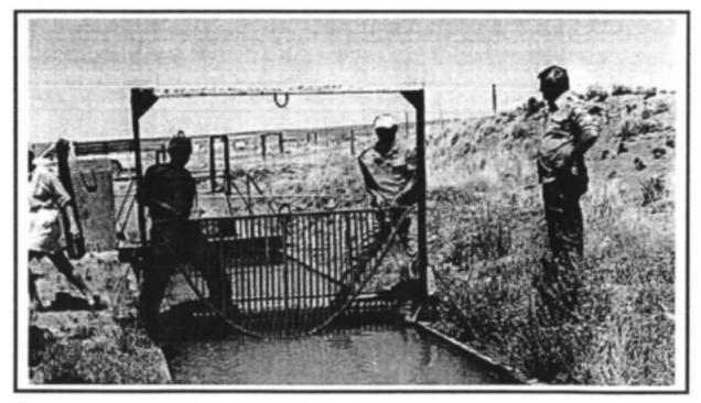
Figure 4.5: A photograph of the vertical bar fish grid used to separate the experimental and control areas.
