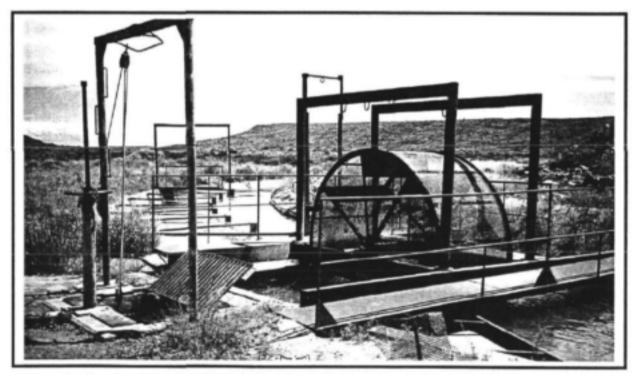
Figure 3.16: An example of a typical roll-grid, in the Ramah Canal System.
