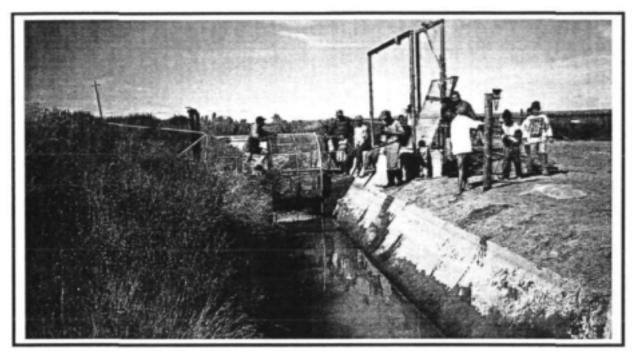
Figure 4.3: A photograph of a typical roll-grid in the Ramah Canal System.
