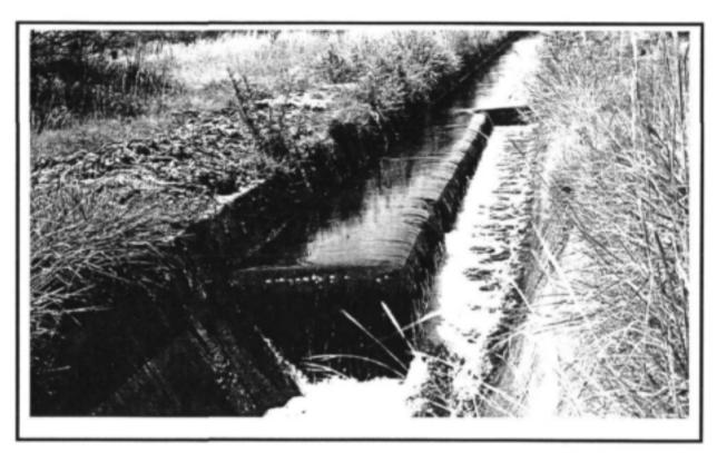
Figure 3.15: An example of a typical long-weir in the Roodeplaat Canal, North of Pretoria.
