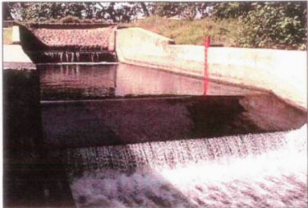
Figure 22 Mzingazi weir W1H011
