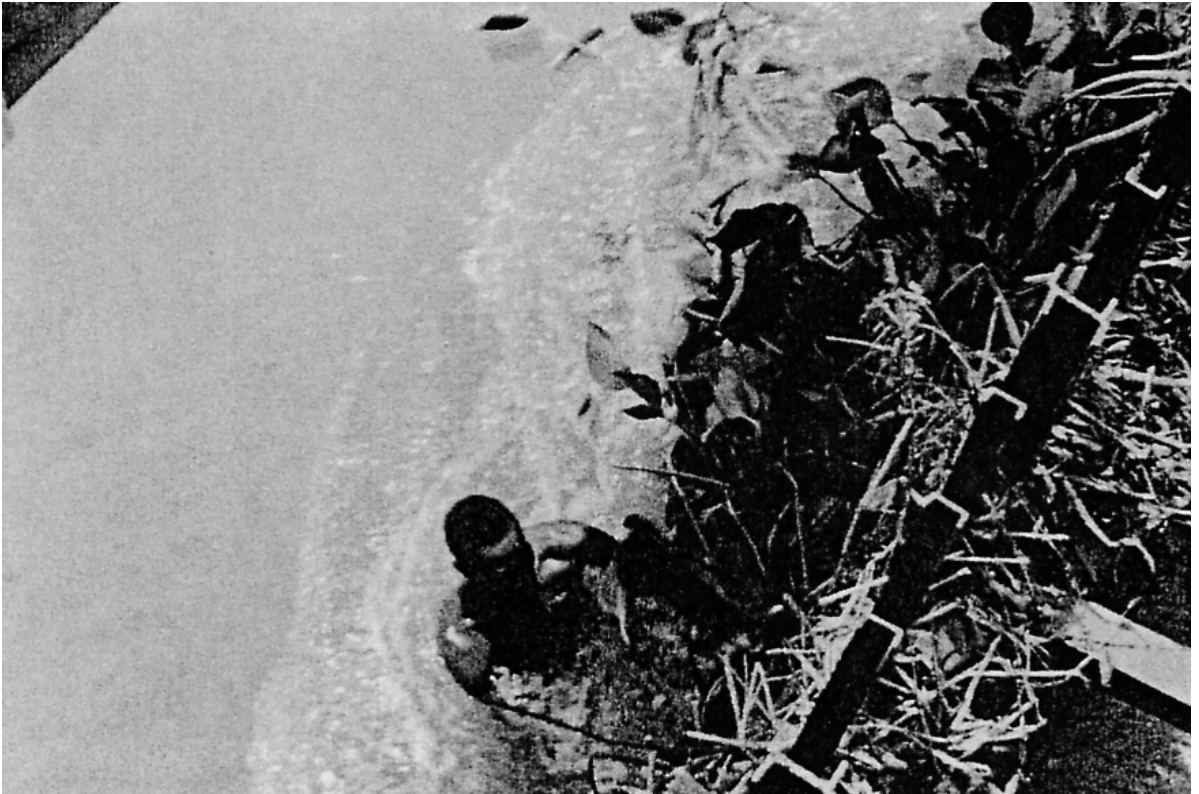
Fig 5.4 (a) Serious clogging of screens by water hyacinths. Niger River, Mali
