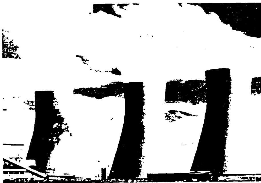
Figure 1.1.9: Natural draft counterflow cooling towers.
