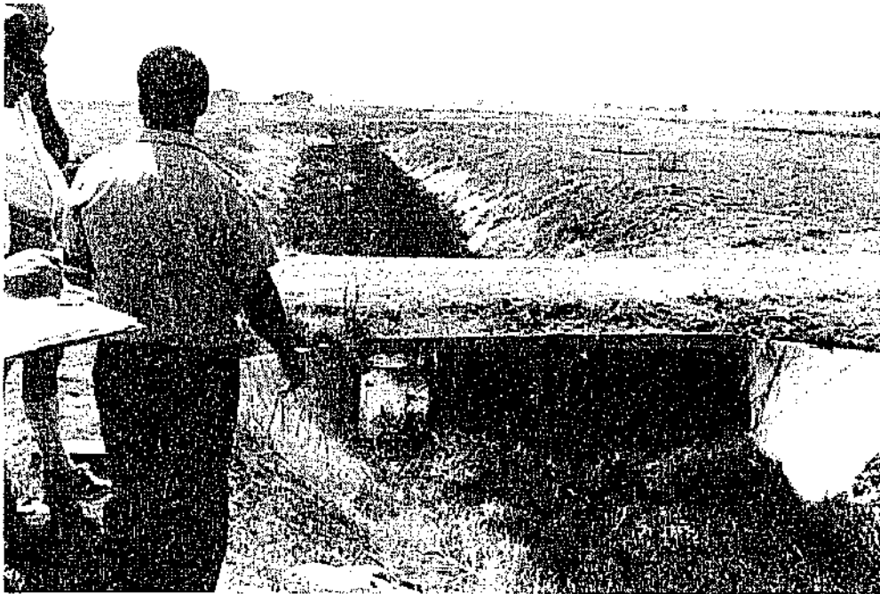
Photo 5 - Grass drainage canal near Mokassa in the Taung area 5/10/92
