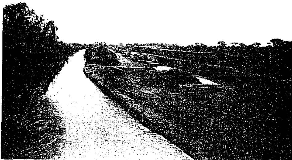
Photo 2 - New canal under construction at Vaalharts Weir 6/10/92
