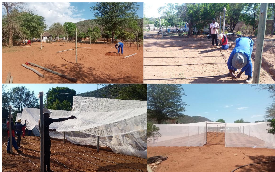
Figure 7.1. Erecting a shade net structure in Lebowakgomo, with irrigation installation.
