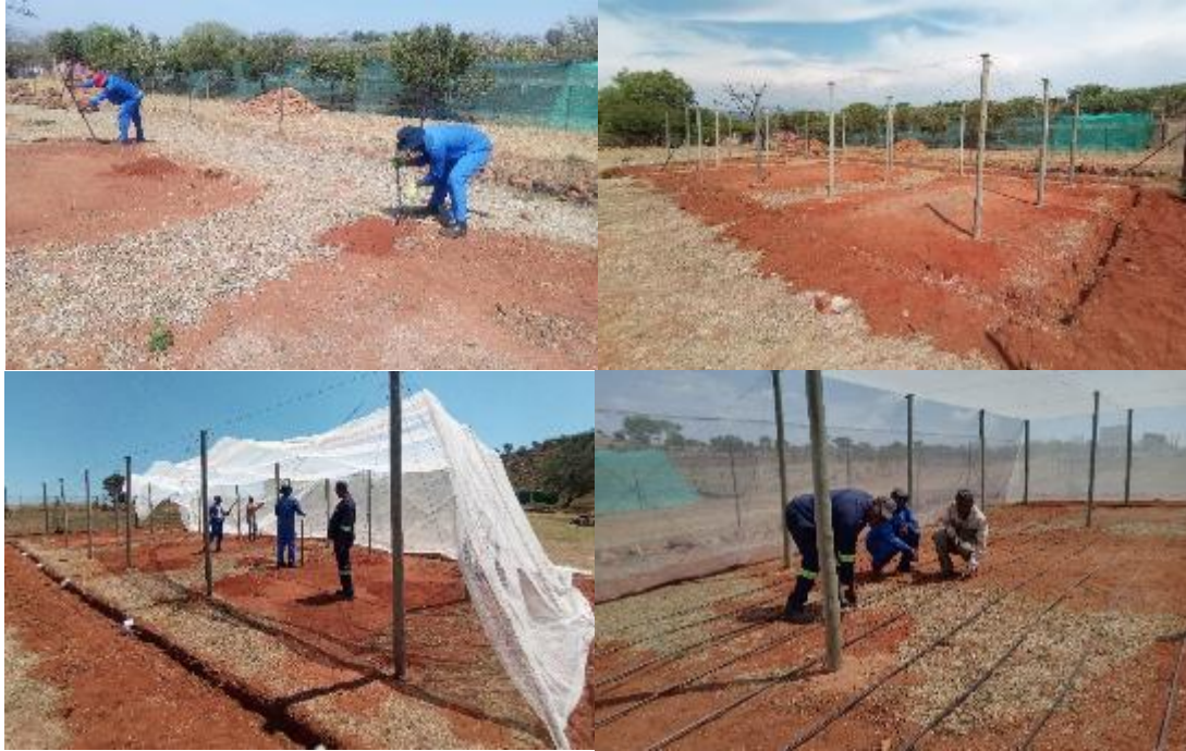
Figure 7.2. Erecting a shade net structure and installing irrigation pipes in Mamelodi.
