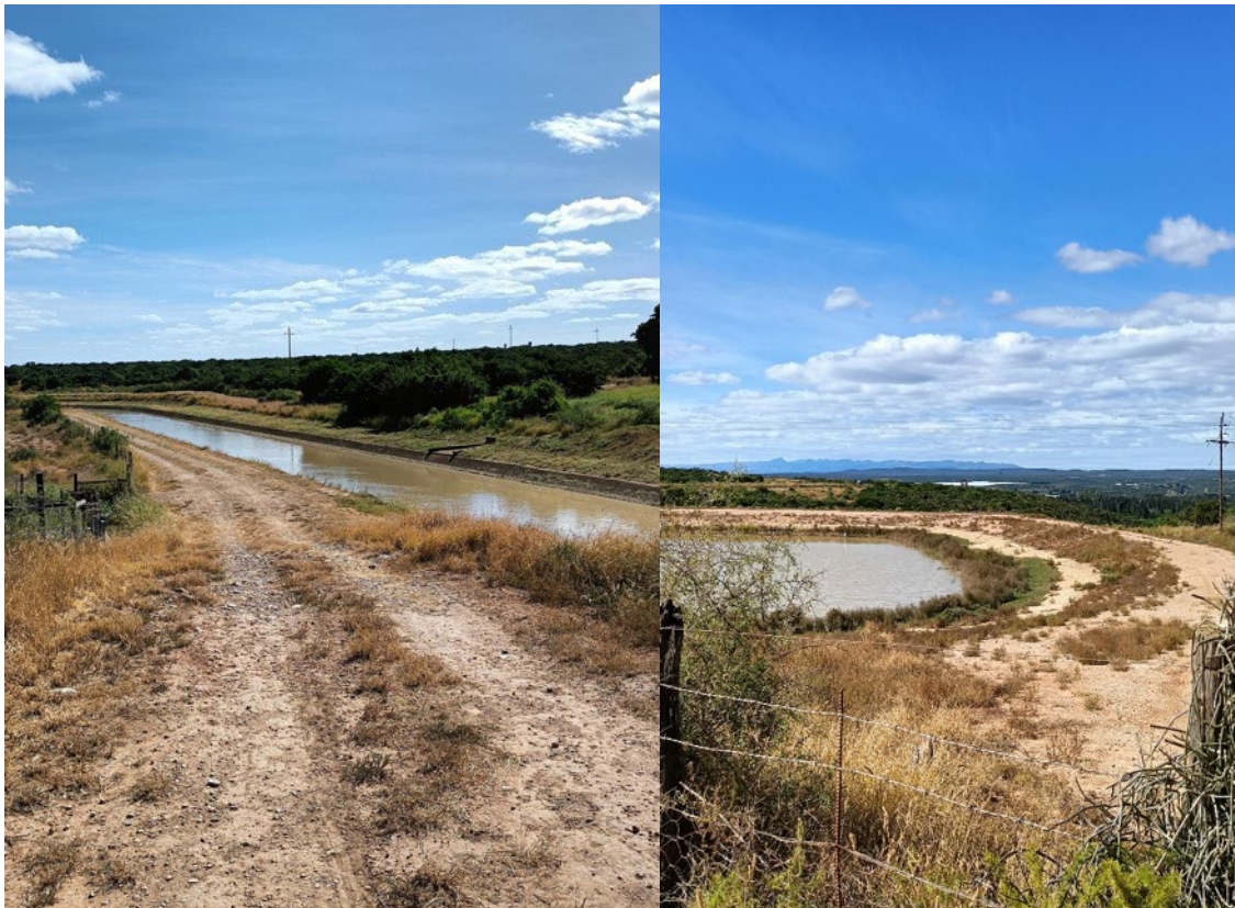
Figure 3: Sections of the Sundays River Canal showing water conveyance infrastructure
