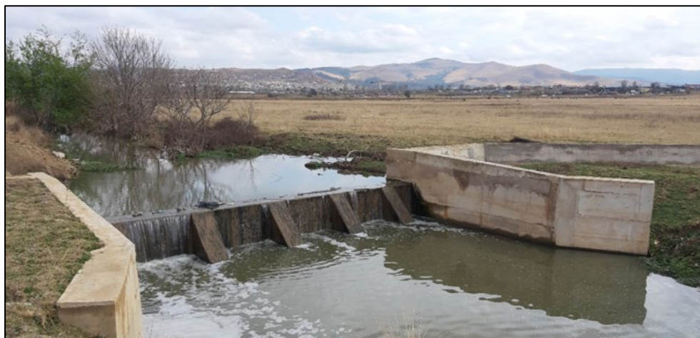
Figure 4-6 Construction of additional weirs in Phase 2 of the uMthinzima Wetland rehabilitation (WfW, 2024)
