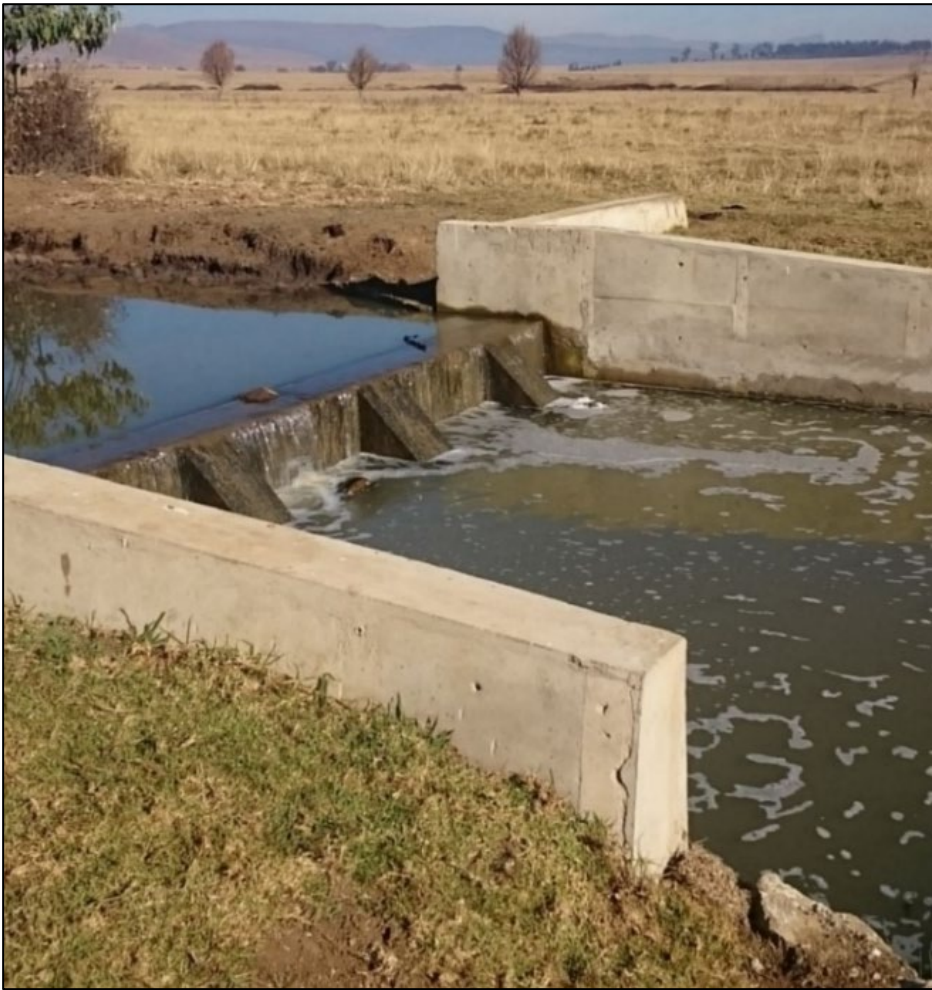
Figure 4-5 Concrete butress weir built during phase 1 of Working for Wetlands construction cycle [source: GroundTruth, June 2019]
