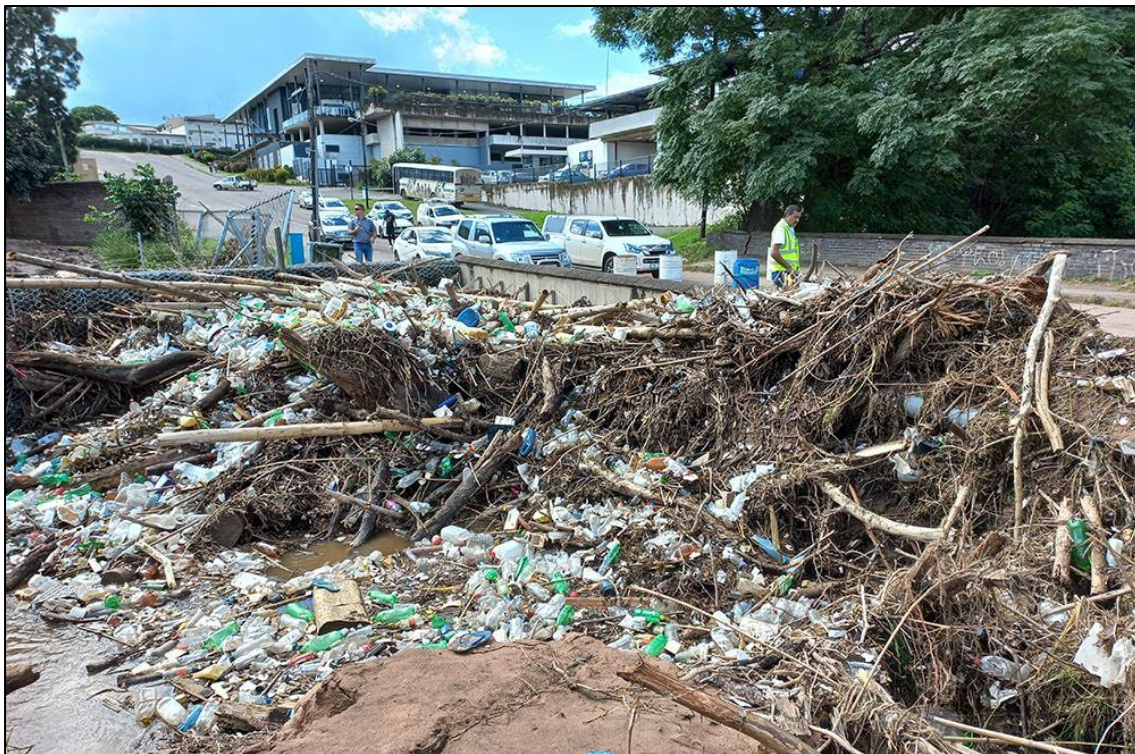
Figure 5-7 Damage to infrastructure and to services adjacent to Caversham Culvert (Durban) during 2022 floods due to blockages being caused by alien vegetation and solid waste (Source: Geoff Tooley, eThekweni Municipality)
