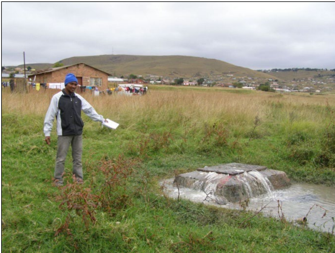
Figure 4-11 One of the Mpophomeni Enviro-Champs pointing at one of the leaking sewer manholes in the Mpophomeni area in 2012 (MSEP, 2013)
