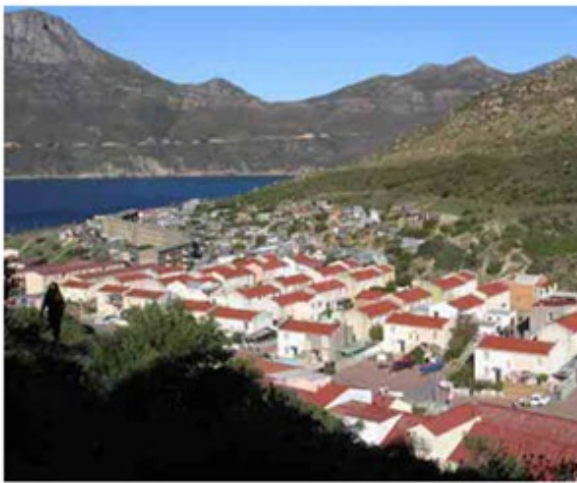
Formal housing (flats) in Hangberg
