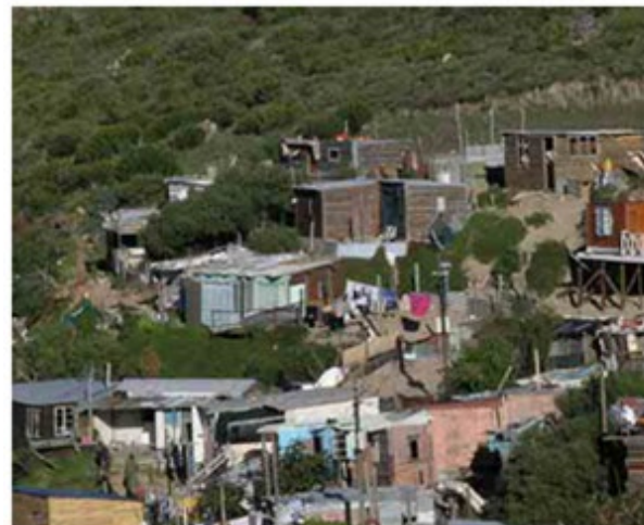
Informal housing in Hangberg
