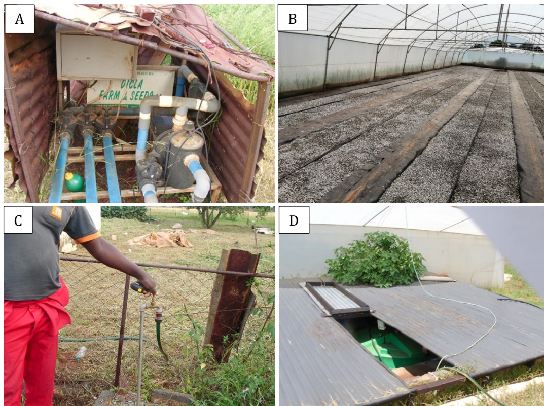
Figure 6.3: Components of the GFT system installed at Mme Mbatha's site: electrical system (a), hydrolines showing a gravity water flow pattern (b), municipal water source (c) and nutrient solution reservoir (d). The system is connected to a 5000-L JoJo tank, which contains a 1.1 kw submersible pump delivering 1650 litres of nutrient solution per hour.
