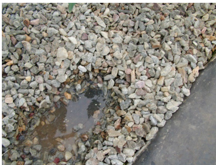
Figure 6.4: Hydroline characteristics: 6 cm deep, covered by 250 micron black plastic at the bottom and filled with 8-13 mm diameter gravel stones.
