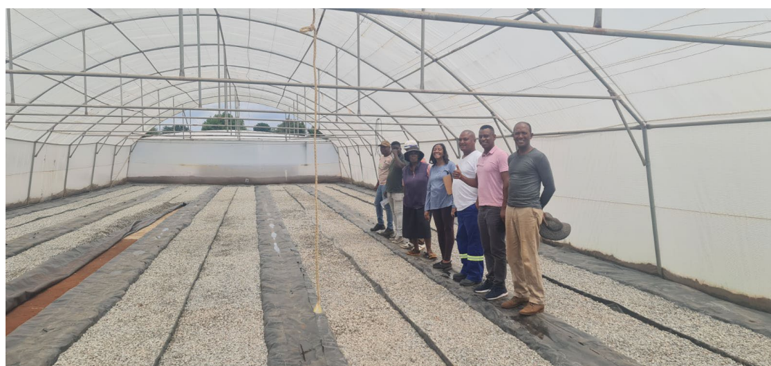
Figure 6.2: A completed GFT system installed at Mme Mbatha trial site in Zuurbekom, West Rand District Municipality. The GFT system uses an electrical
