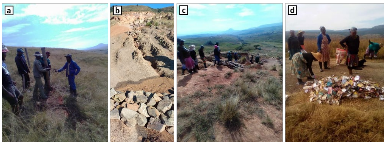
Figure 8-4 Costone. a: Grazing management (moving gate and fixing fence line of grazing camp), b-c: erosion control (community members constructing check dams and stone packs), d: river cleaning (A group of women spent a day collecting waste that was discarded in water courses in the community)
