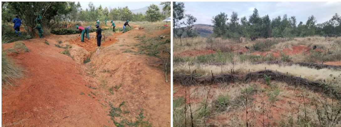
Figure 8-3 Wattle clearing, brush packing and planting of grass for erosion control in Costone
