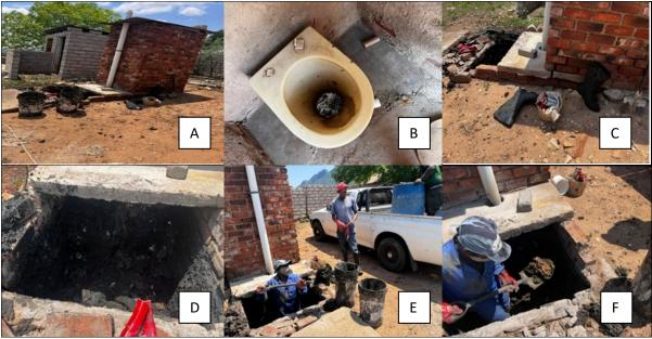
Figure 9-12: Process of cleaning the pit latrines
