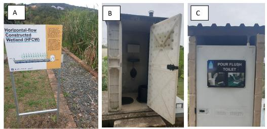
Figure 9-13: Decentralised sanitation toilets and treatment system at Newlands-Mashu research station: A: Horizontal flow constructed wetland; B: Urine diversion toilet; C: Pour flush toilet
