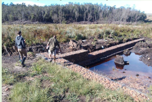
Figure 4: An example of wetland rehabilitation gabion structure constructed by Working for wetland. These structures require regular monitoring to measure their impact on restoring the wetland functions.
