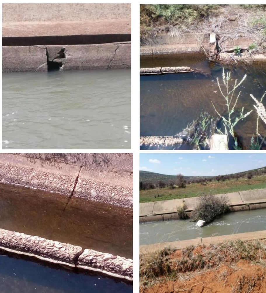
Figure 1: Photos illustrating the condition of some sections of the canals at Vaalharts and Loskop irrigation schemes. Sections showing deteriorated conditions were found across all canal levels, i.e. main, secondary and tertiary canals.
