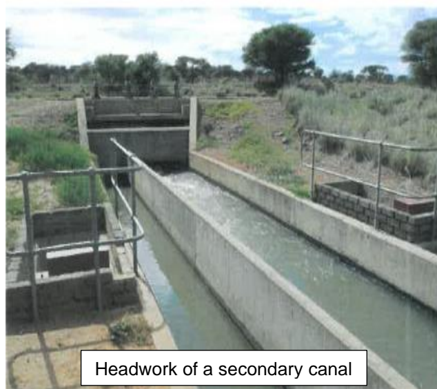
Offtake point from a main canal section
