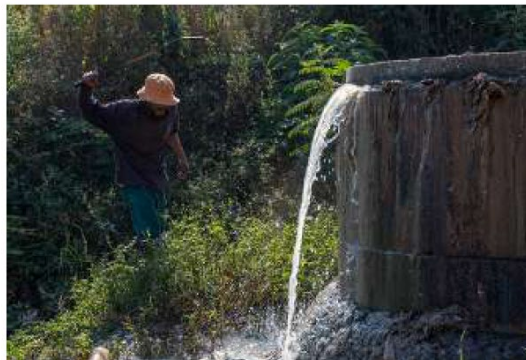
A MEMBER OF THE DUCT SEWER MONITORING TEAM CLEARING THE AREA AROUND A LEAKING MANHOLE
