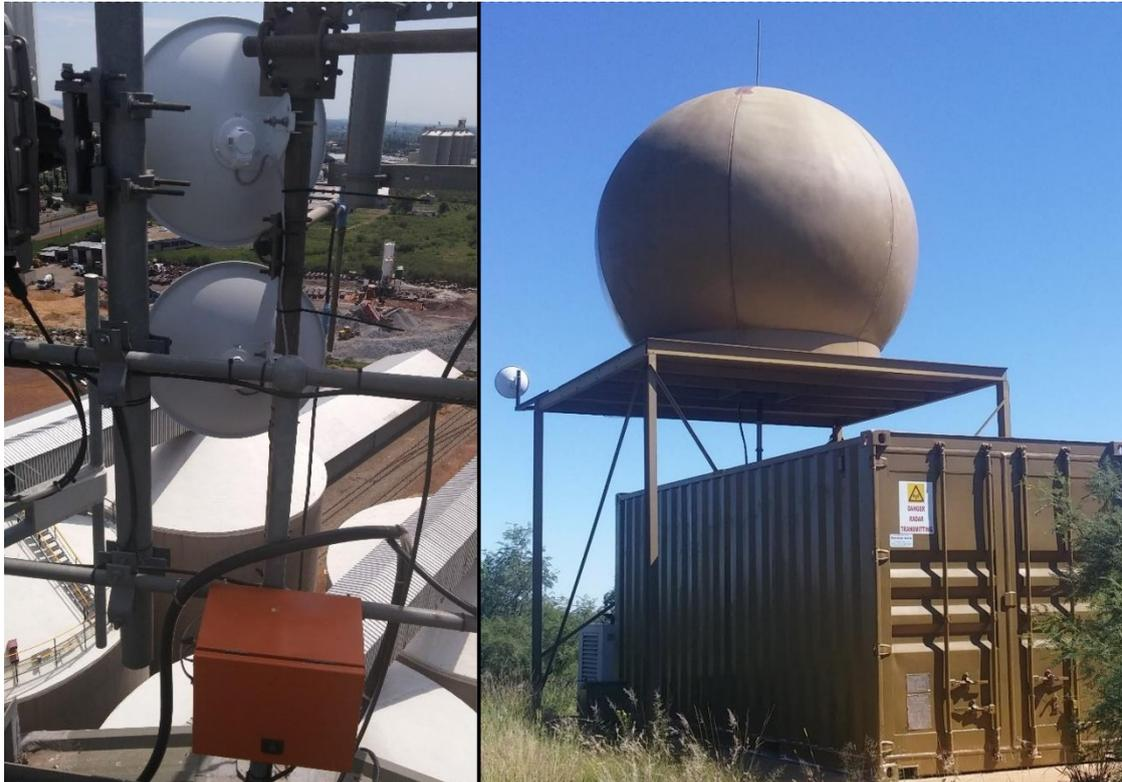
**Figure 4.12: The first radio link established between the radar and NWU. The photograph on the left shows the antennae on the silos and the photograph on the right shows the antennae on the radar.**
