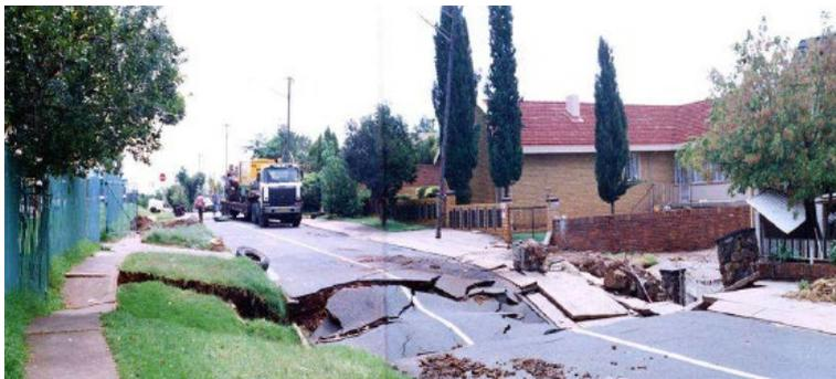
Figure 2-6: Damage to houses in Laudium in Pretoria due to a sinkhole (Oosthuizen and Richardson, 2011)
