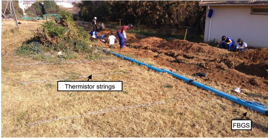
Figure 3-13: Sensor layout and levelling bottom of trench in preparation for pipe and instrumentation installation
