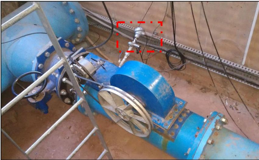
Figure 3-6: RTD installed at Pierre van Ryneveld reservoir
