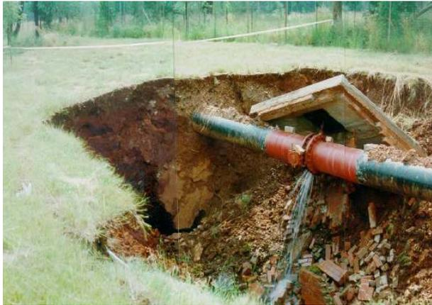
*Figure 2-7: Leaking water pipe caused a sinkhole to form in Waterkloof, Pretoria (Oosthuizen and Richardson, 2011)*
