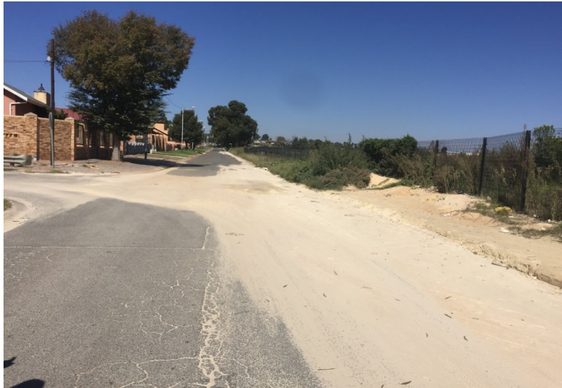
Figure 3-16 Tailings dump material eroded to the streets.
