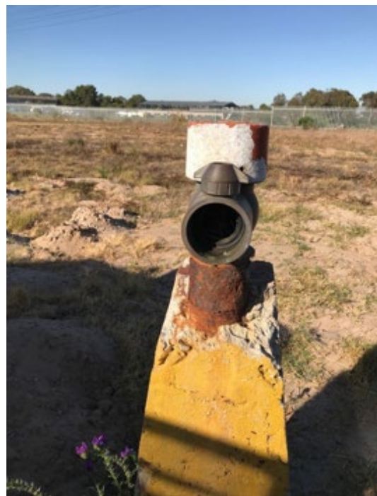
Figure 4.33: Fire hydrant connection
