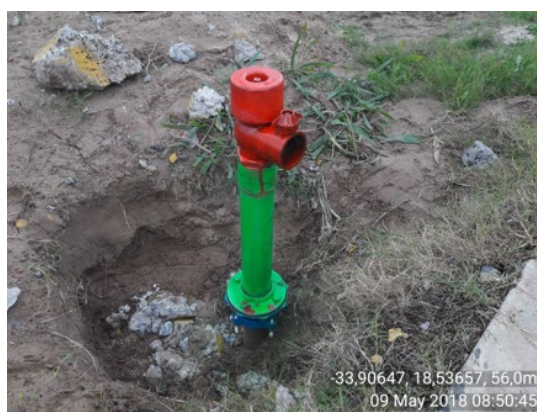
Figure 4.35: The replaced fire hydrant pipe with the hydrant head
