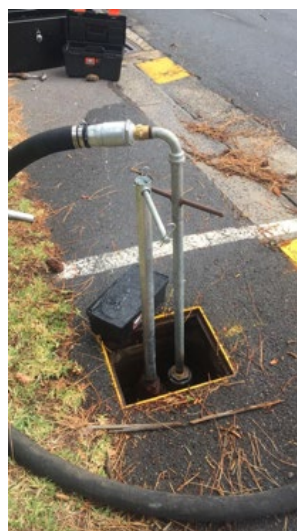
Figure 4.41: Underground fire hydrant connection
