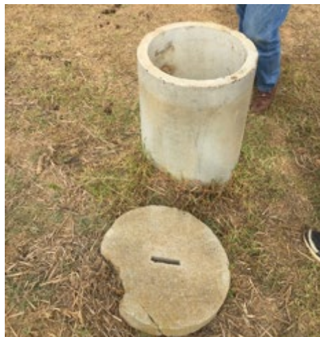
Figure 4.4: The air valve's concrete chamber
