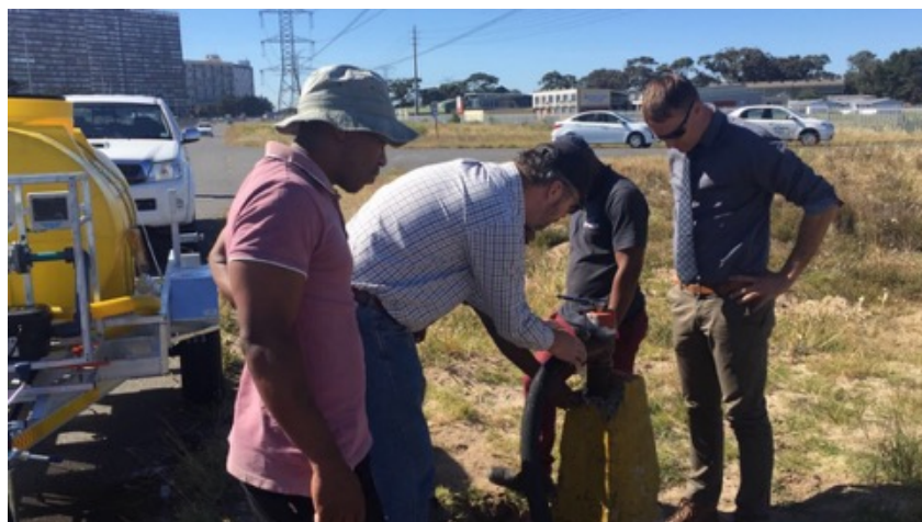
Figure 4.23: Black 50 mm hosepipe being connected to the fire hydrant
