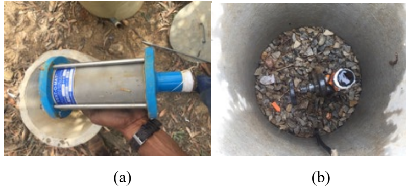
Figure 4.5: (a) The air valve; and (b) the BS 8 pipeline stop valve connection
