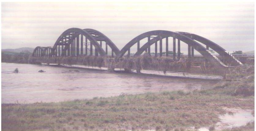
Photograph 2-5: Photograph of the old N2 Road Bridge several hours after the main flood peak had receded following an approximate 1:100 year rainfall event in September 1987. (Photo Kelbe)
