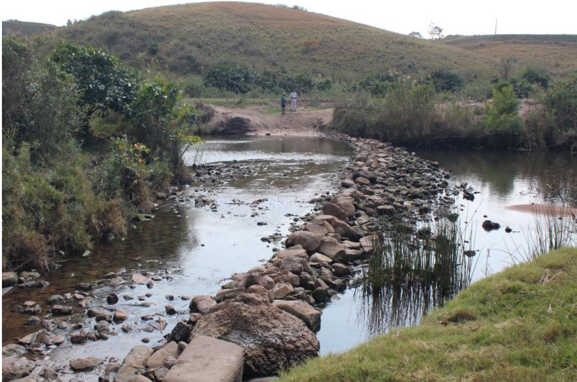
**Figure 6-2:** The road-crossing in the upper portion of the Mlalazi Estuary. High tides rise above the rocks to flood the tributary area upstream of this causeway. (Photo R Taylor, 28 August 2012).
