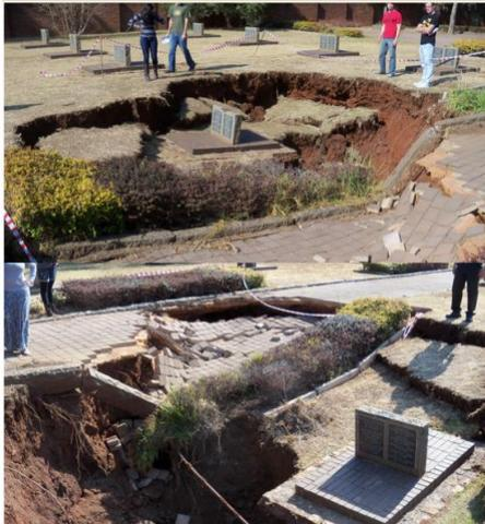
(left) Dolomite in the Irene Cemetery (2012): a leaking water pipe mobilised overburden into a sinkhole through the ingress scenario. Landscaping and irrigation were the anthropogenic causes of the sinkhole.
