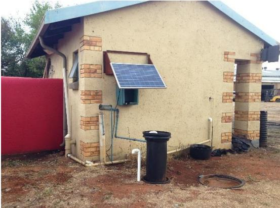
Recycling flush water system with solar panel
