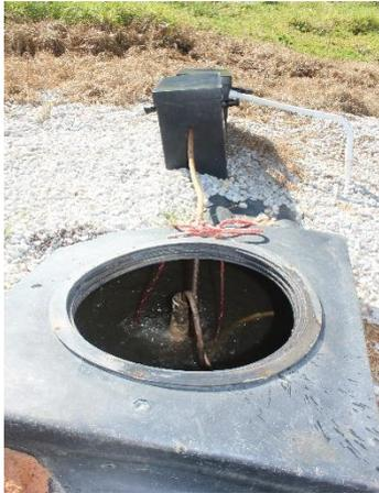
Inlet into first chamber with 12V pump
