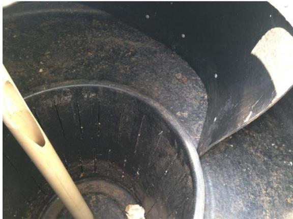
**Image of the turntable and sump basket, with the directional wall for directing faeces into the basket**
