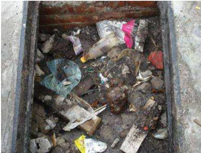
Figure 7-5: Meter chamber filled with rubbish (De Bruyn, 2009)
