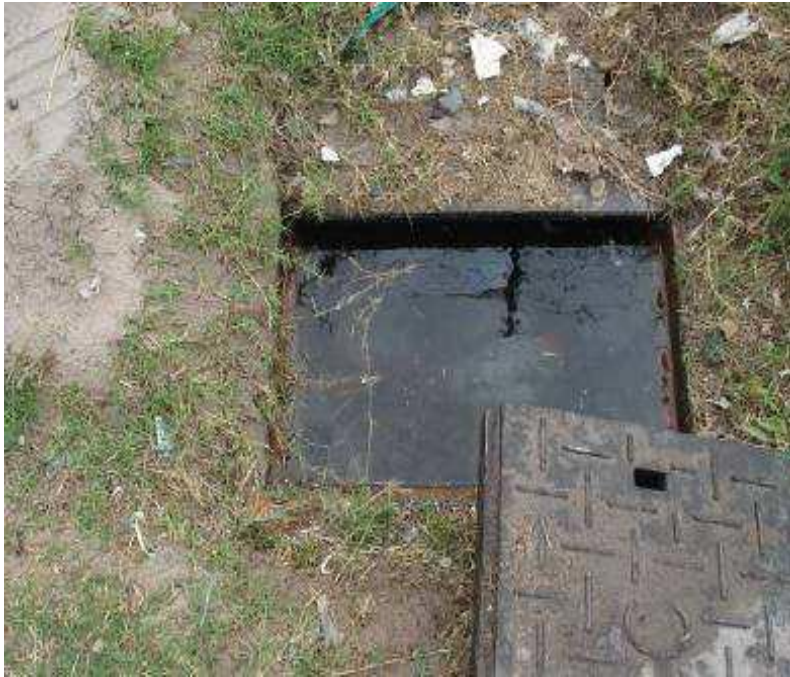
Figure 7-4: Flooded meter chamber (De Bruyn, 2009)
