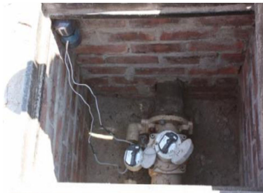
Figure 7-2: Actaris Combination meter with two-channel MIU (De Beer, 2010)
