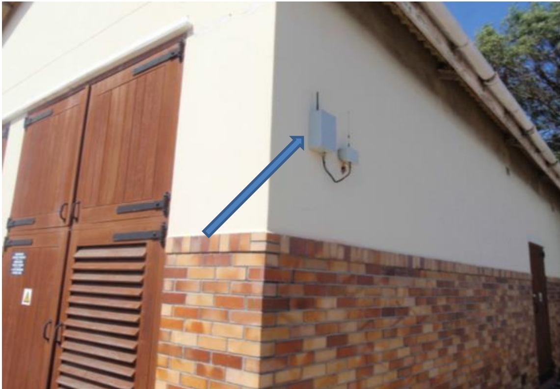
Figure 7-3: GSM unit mounted with Isolating switch (De Beer, 2010)
