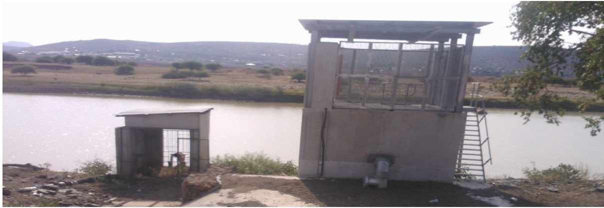
Figure 4.8. The electric generator pump station in Block 4B
