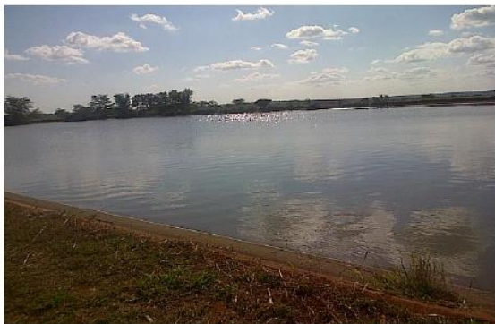
(a) Canal dam
