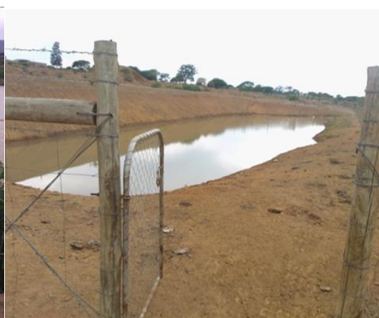
b. Smaller dam supplying blocks 3 and 4
