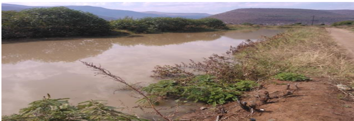
Figure 4.11. The dam for Block 4B
