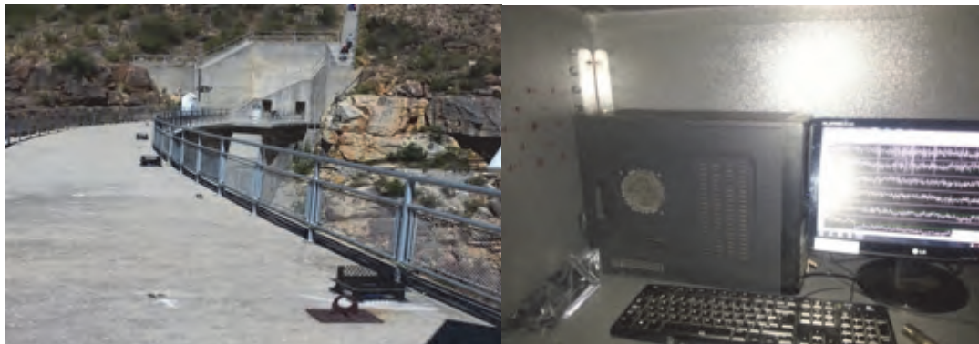
Figure 4.1: Accelerometers on the dam crest and data acquisition system in the upper dam gallery
