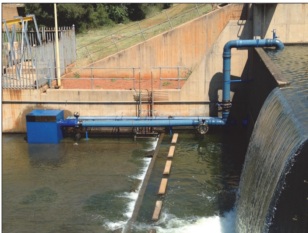
Figure 9-52: Zeekoegat WWTW - Low Head hydropower installation
