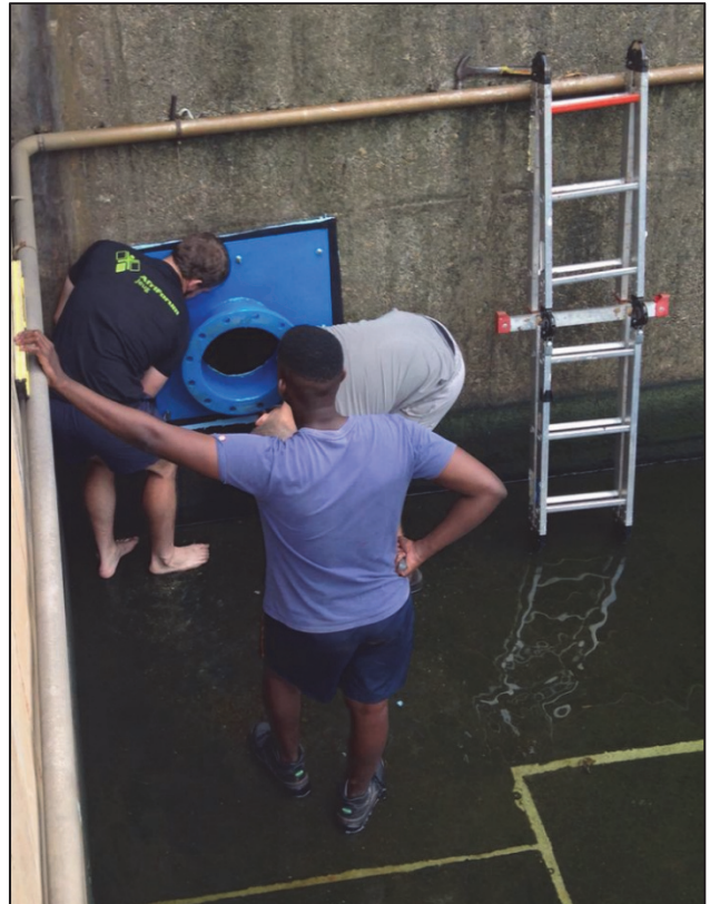
Figure 9-35: Installing the offtake plate against dam wall
