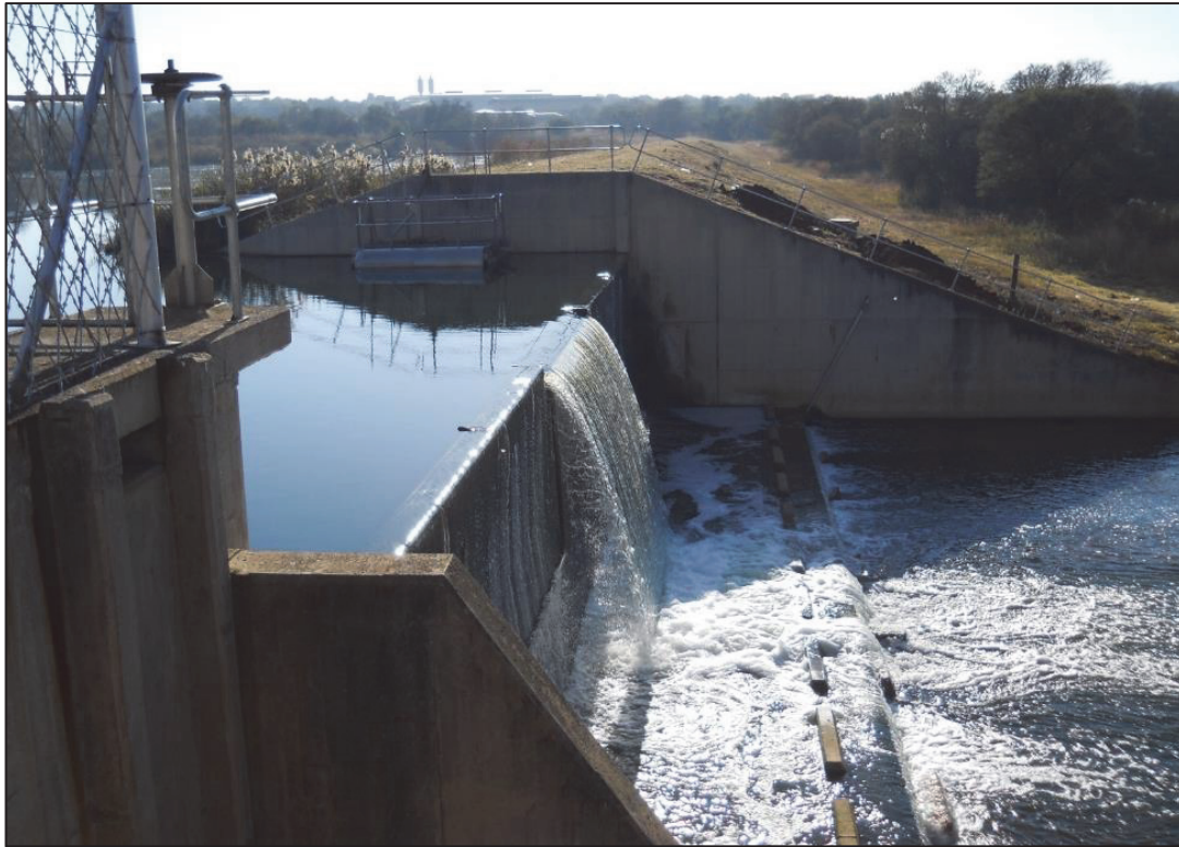
Figure 9-3: Zeekoegat WWTW outlet structure
