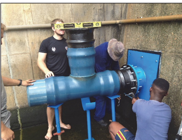
Figure 9-39: Connection to existing scour point
