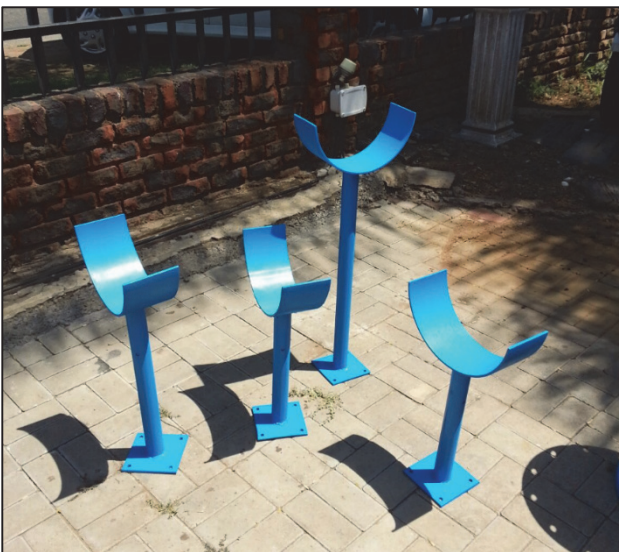
Figure 9-34: Constructed pipe supports
