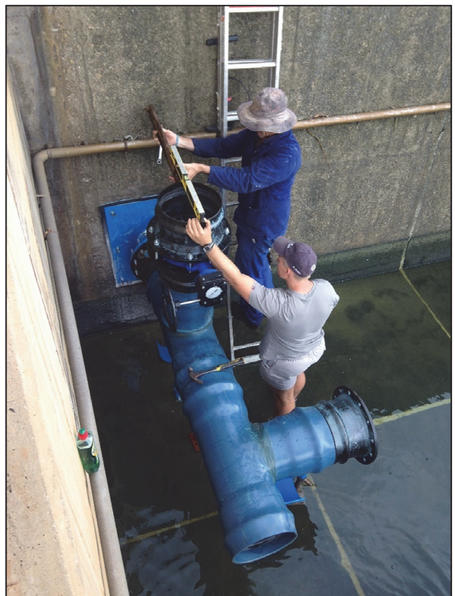
Figure 9-41: Measurements for connecting siphon
