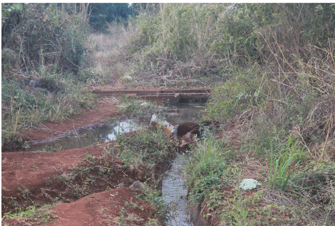
FIGURE 7.3: Water leaking from the main canal diverted to Mashudu’s ‘wasteland’ plot
