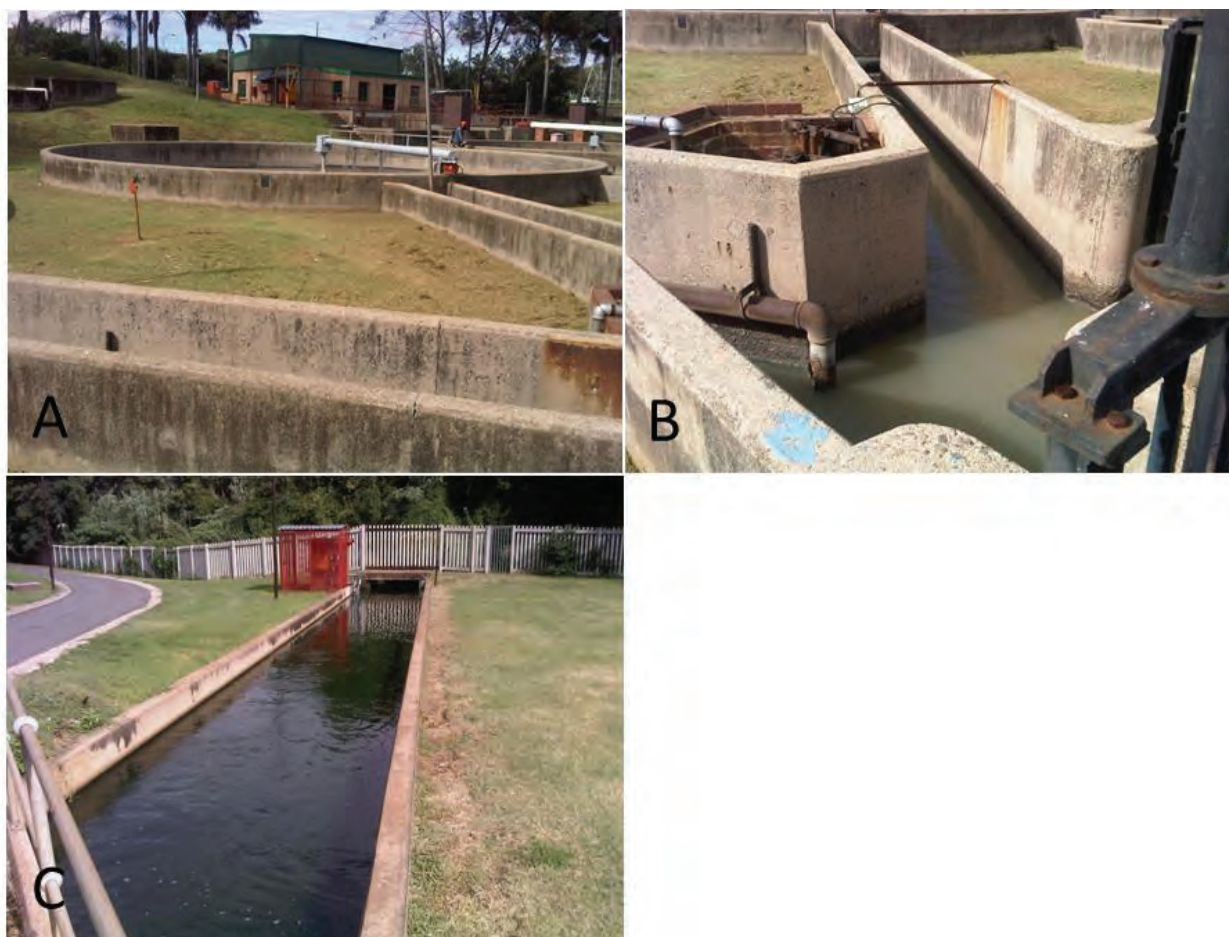
Figure 4-2: Daspooort sampling points; A & B show influent sampling point #2 and C is effluent sampling point
