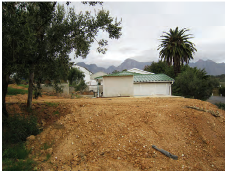
Figure 6: Site preparation for the container and external tanks. The concrete building in the background stands on top of the factory wastewater sump
