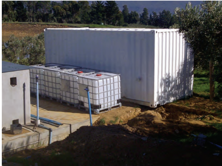
Figure 10: Tank installation and earthworks for piping
