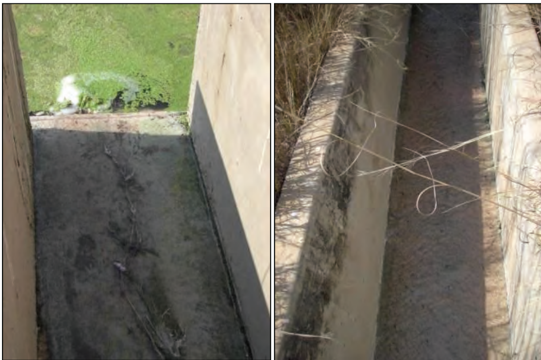
Figure 2-79: Elemental sulphur, an oxidation product of hydrogen sulphide, precipitates on the overflow weirs of duckweed-based maturation ponds
