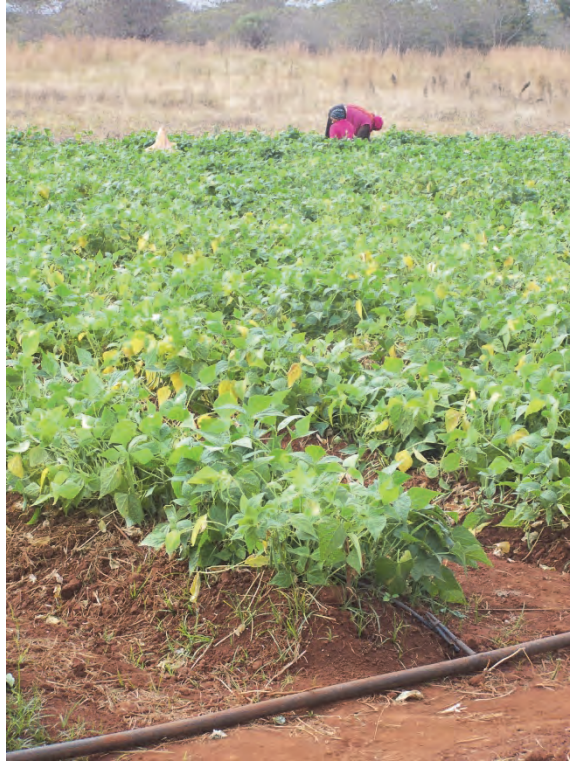
Photograph 16: Drip irrigation system (respondent F)
