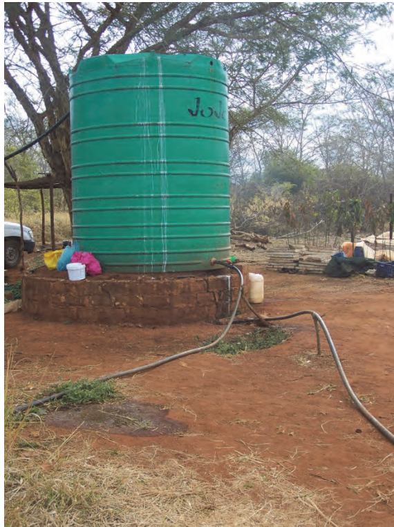
Photograph 17: Inadequate storage (respondent F)
