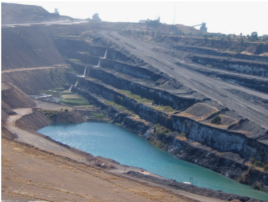
Figure 160: An obsolete sump being backfilled (courtesy of the Grootegeluk mine).
