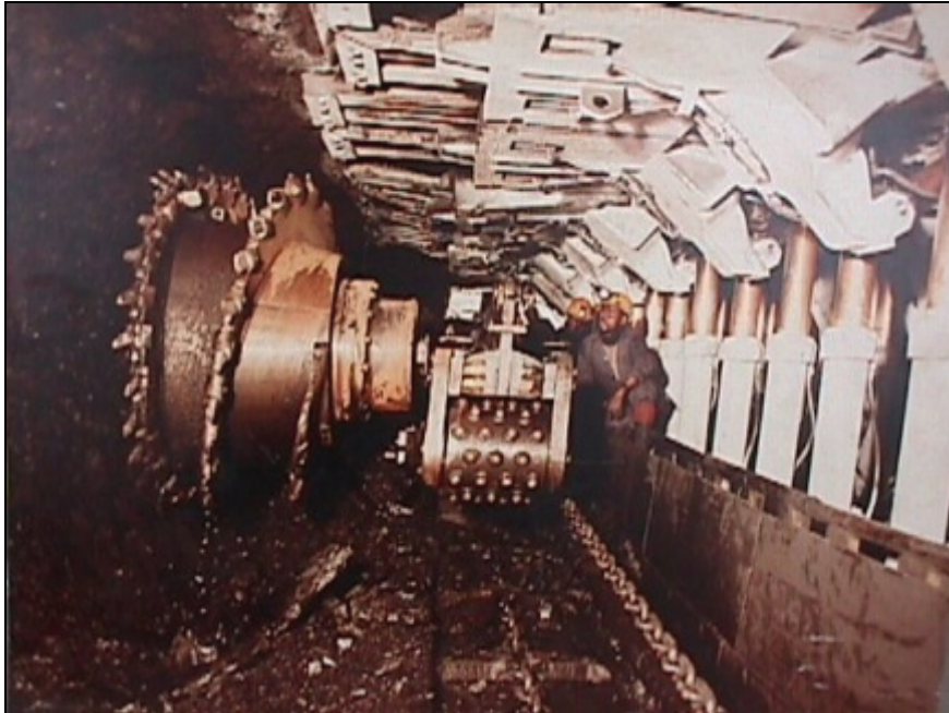
Figure 9: A longwall mining operation (Grobbelaar, 2001).
