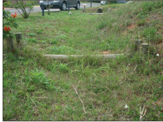
Figure 4-31: Wooden weir to capture smaller objects in Hawaan Estate
