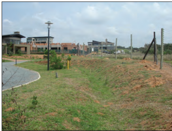
Figure 4-32: Access road linked to a vegetated swale in Hawaan Estate
