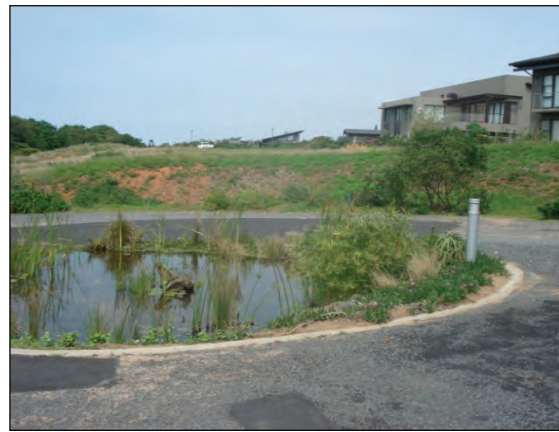
Figure 4-33: Small retention pond at the end of an access road in Hawaan Estate
