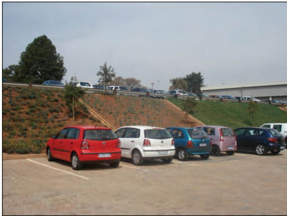
Figure 4-8: Embankment separating the two Wits parking areas (above)
