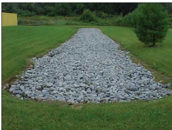
Figure 2-6: Infiltration trench servicing a gated village
