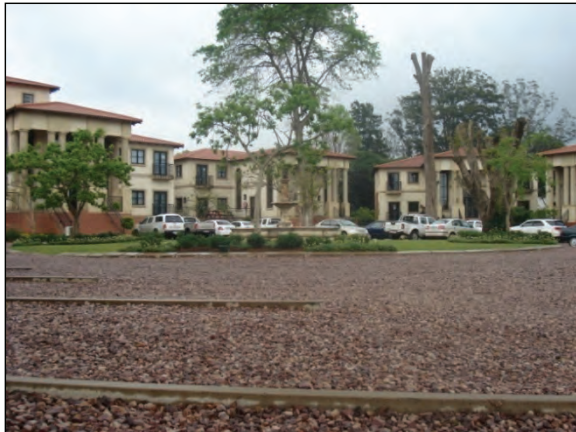
Figure 4-16: Multi-coloured aggregate used for parking bays
