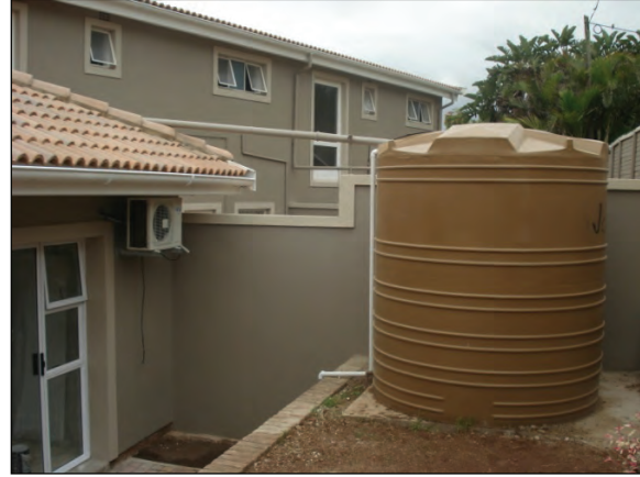
Figure 2-5: Rainwater harvesting tank, Selborne Estate, East London
