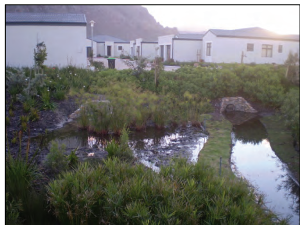
Figure 2-7: Bio-retention area underlying footbridge, Evergreen Retirement Village, Cape Town
