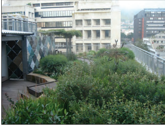
Figure 2-4: Intensive green roof, CBD, Cape Town
