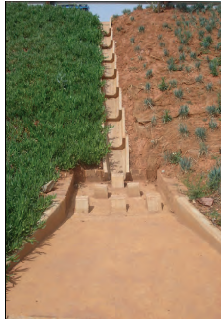
Figure 4-9: Chute and energy dissipater on the Wits embankment (right)
