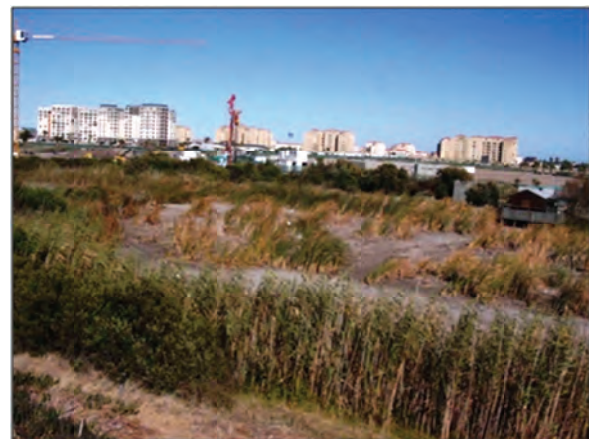
Figure 4-40: Cell 2 during the wetland's construction phase
