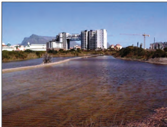
Figure 4-39: Cell 1 after routine dredging
