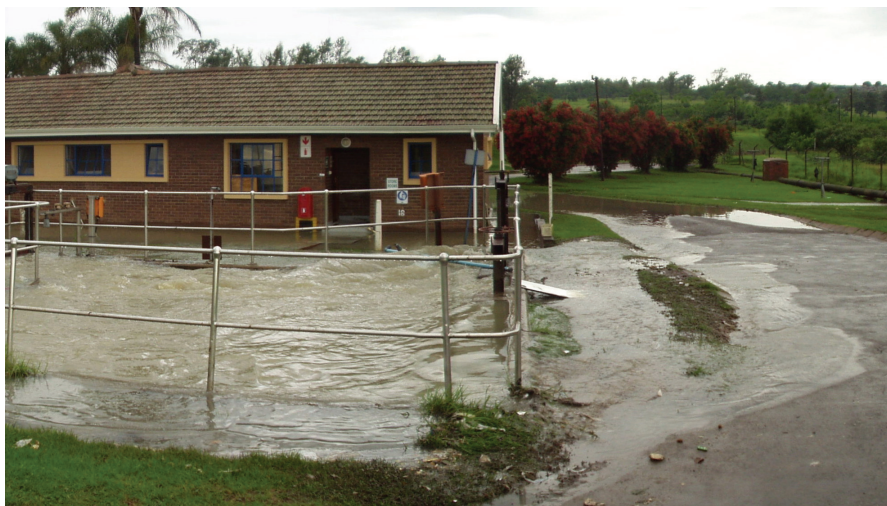
Figure 2: Darvill Waste Water Treatment Works overflowing during a storm in Pietermaritzburg (Steve Terry, 2007)
