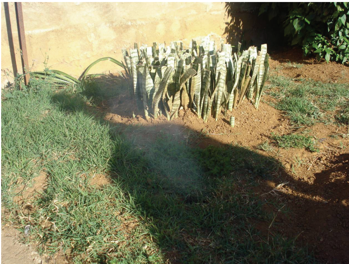
Figure A4: Smoke rises from the ground in a patch of lawn, revealing a broken sewer pipe below the surface. As with the break shown in Figure A3, a problem like this would be hard to find using a routine visual inspection.
