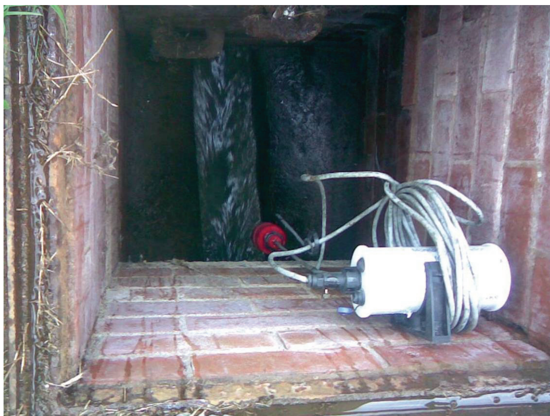
Figure 32: Installation of sewer flow logging equipment at Ward 31 site
