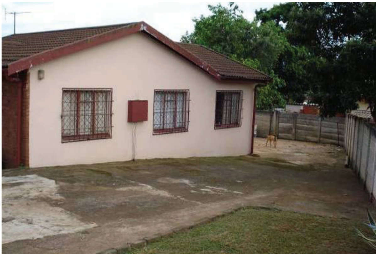
Figure 21: A typical yard in the Northdale area, with a large percentage paved and the downpipes disappearing into gullies which may be connected to the sewer network.
