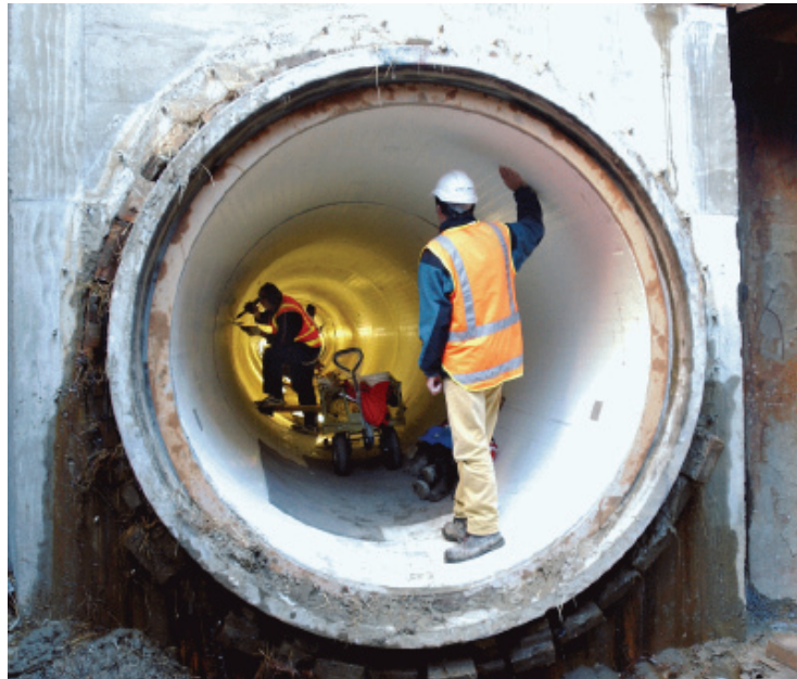
Figure 15: Construction of the Browns Bay on line storage tunnel (Source: Wisumperuma and Vercruyssen, 2006)
