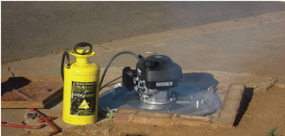
Figure A2: The smoke machine in place over a manhole and in operation. A base plate adaptor is needed to enable the machine to work more effectively over manhole openings (such as this one) which are not an exact match for the machine's base plate.
