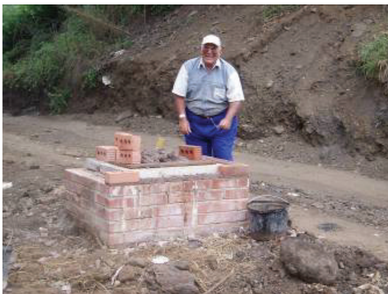
Figure 14: “Vandal proof” manhole covers
