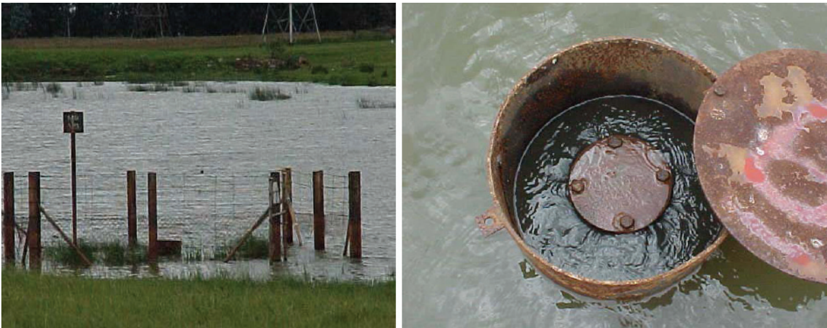
Figure 22: Dam with surface run-off and recharge borehole from the dam into the mine
