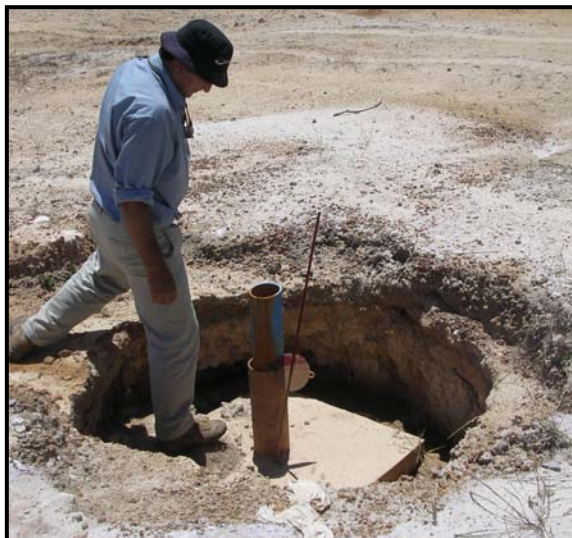
Boreholes must be properly completed to avoid collapse and prevent posing a threat to man and the environment.
