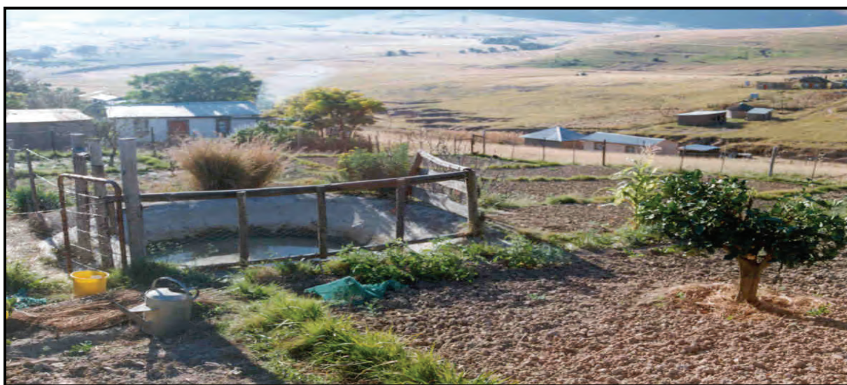
Figure 3.4 Small dam constructed from soil, and lined with cement provides irrigation for home gardening.
