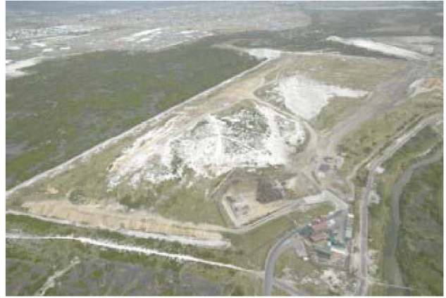
Figure 6.8: The Coastal Park waste disposal site
