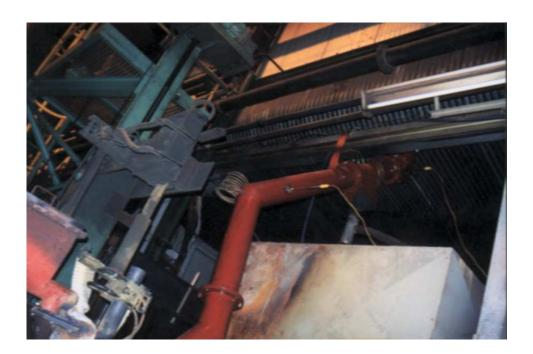
Figure 5.9: Off-gas line with wet scrubber
