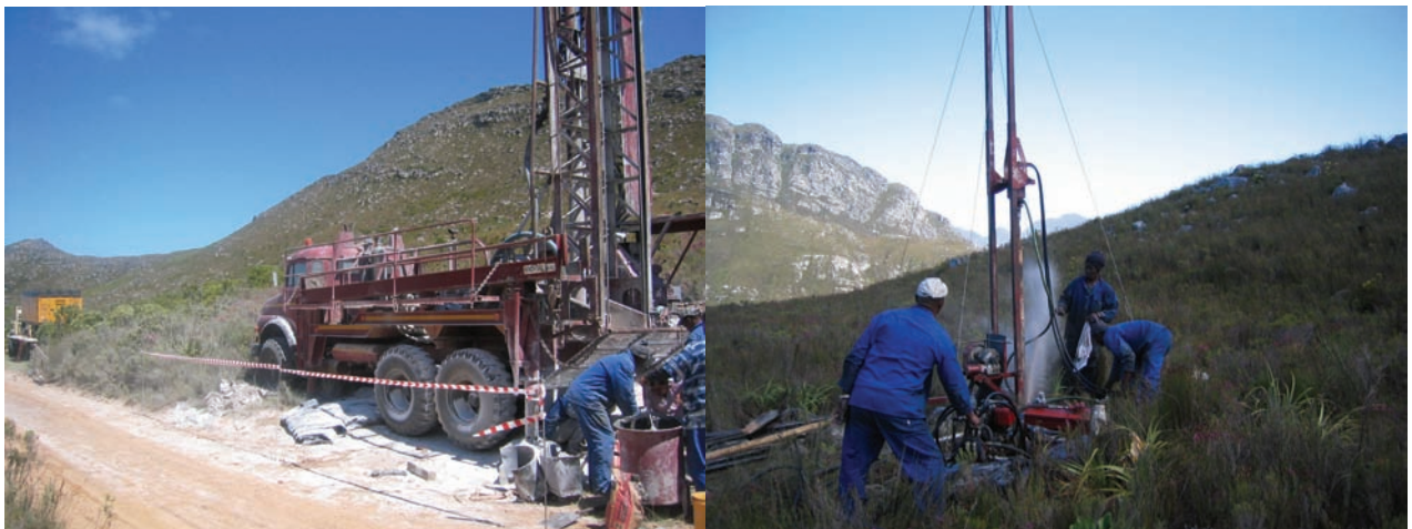
Figure 2-2 Drilling at Kogelberg with the standard 'down the hole' hammer rig (left) and the portable rig (right)
