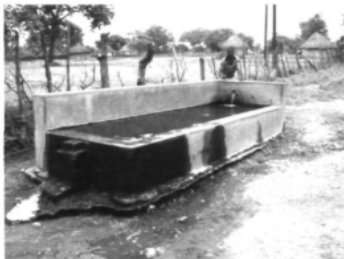
Figure 19: Deionization plant brine discharge point
