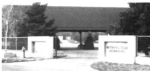
Figure B1 Bisamberg in-situ denitrification plant
