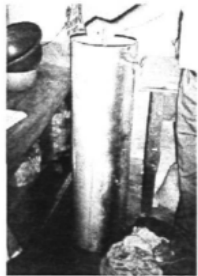
Sri Lanka – a typical domestic unit as installed in a home.
