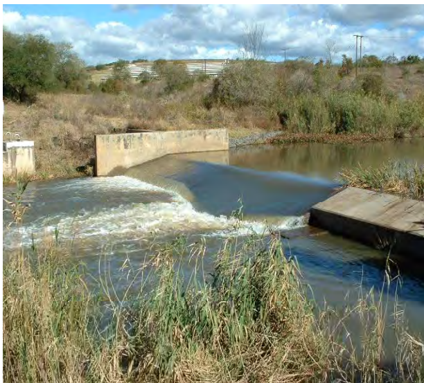
MLAAS ROAD WEIR STREAM GAUGE
