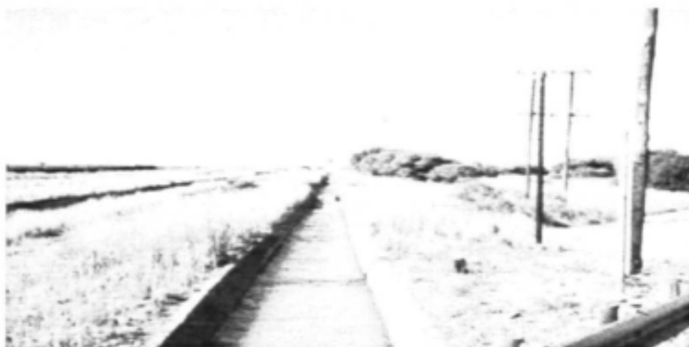
Photo 3.2 Main irrigation canal system used for water distribution at Riet River irrigation scheme
