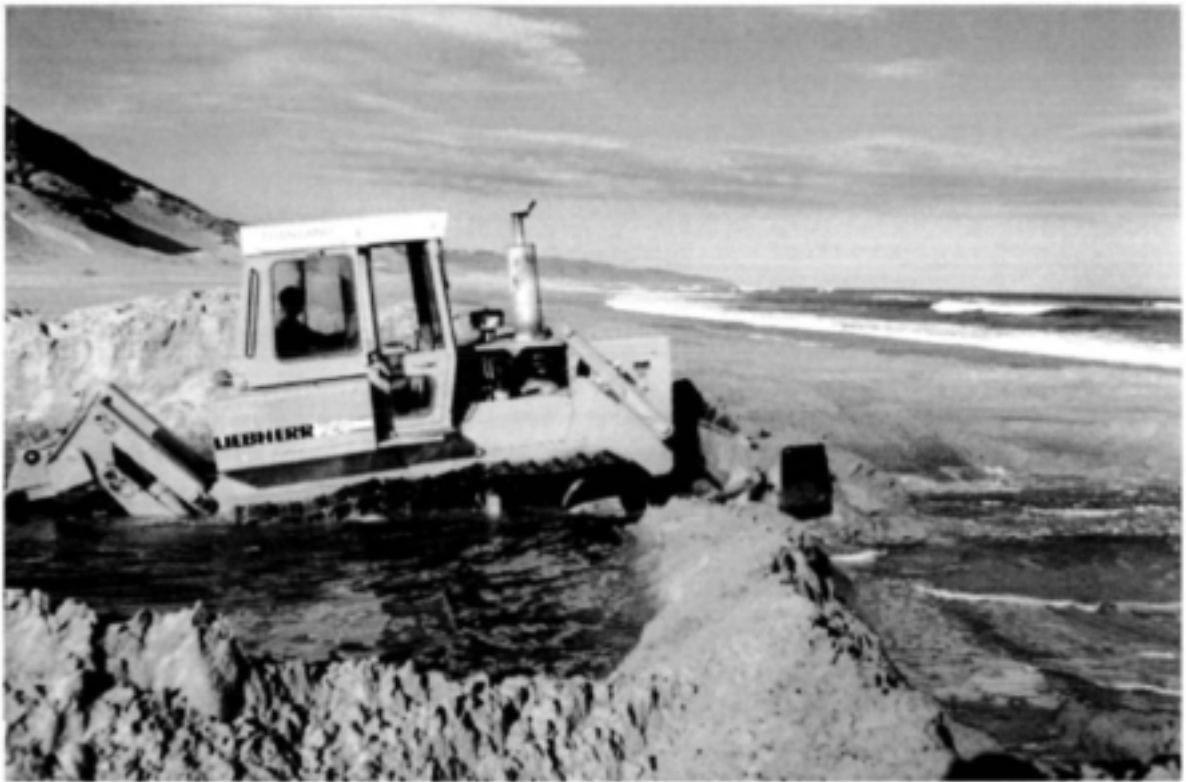
Figure 3.1 Breaching the mouth of the Great Brak Estuary using a bulldozer (Photo: P Huizinga)
