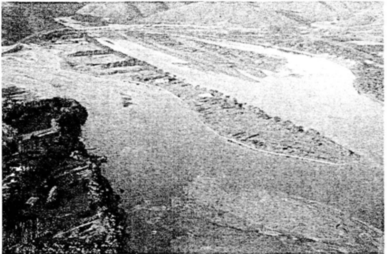
Figure 2.5 The change in estuarine landscape in the Keurbooms Estuary from a confined drowned-valley situation landward of the N2 road bridge (top left in photo) to an open floodplain condition seaward of the bridge. The lack of flow confinement has caused deposition of sediment bodies, called bayhead deltas, during river floods. Such unconfined flow is much less effective in naturally scouring sediment from affected estuaries than confined flow. The channel in the foreground is the much smaller Bitou Estuary tributary that joins the Keurbooms Estuary at the right of the photograph. (Photo: J S V Reddering)
