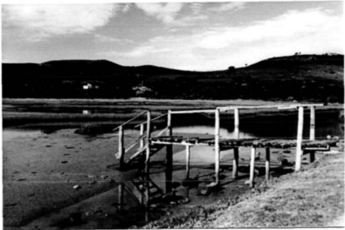
Figure 3.2 A jetty left high and dry by sedimentation processes near Leisure Island in the Knysna Estuary. (Photo: P Huizinga)
