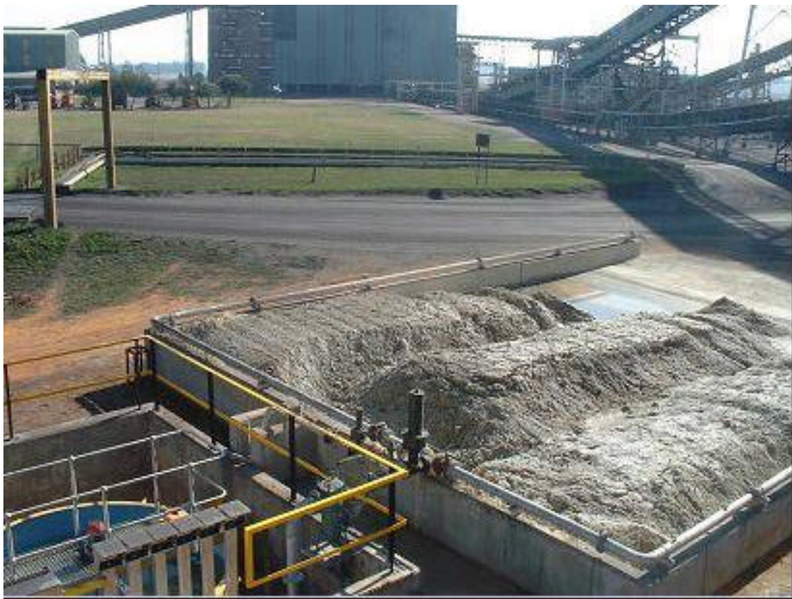
Figure 9.1 Limestone handling and dosing system.
