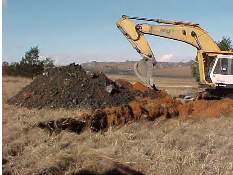
Figure 86. Excavator and removed spoils in an inspection pit.
