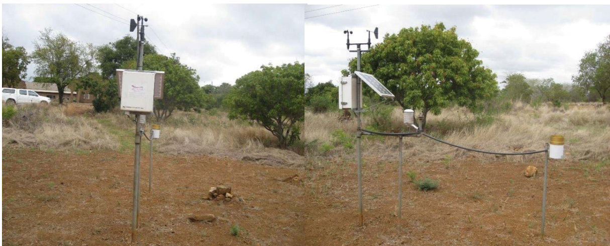
Figure 4: Installed weather station at Malamulele agricultural offices
