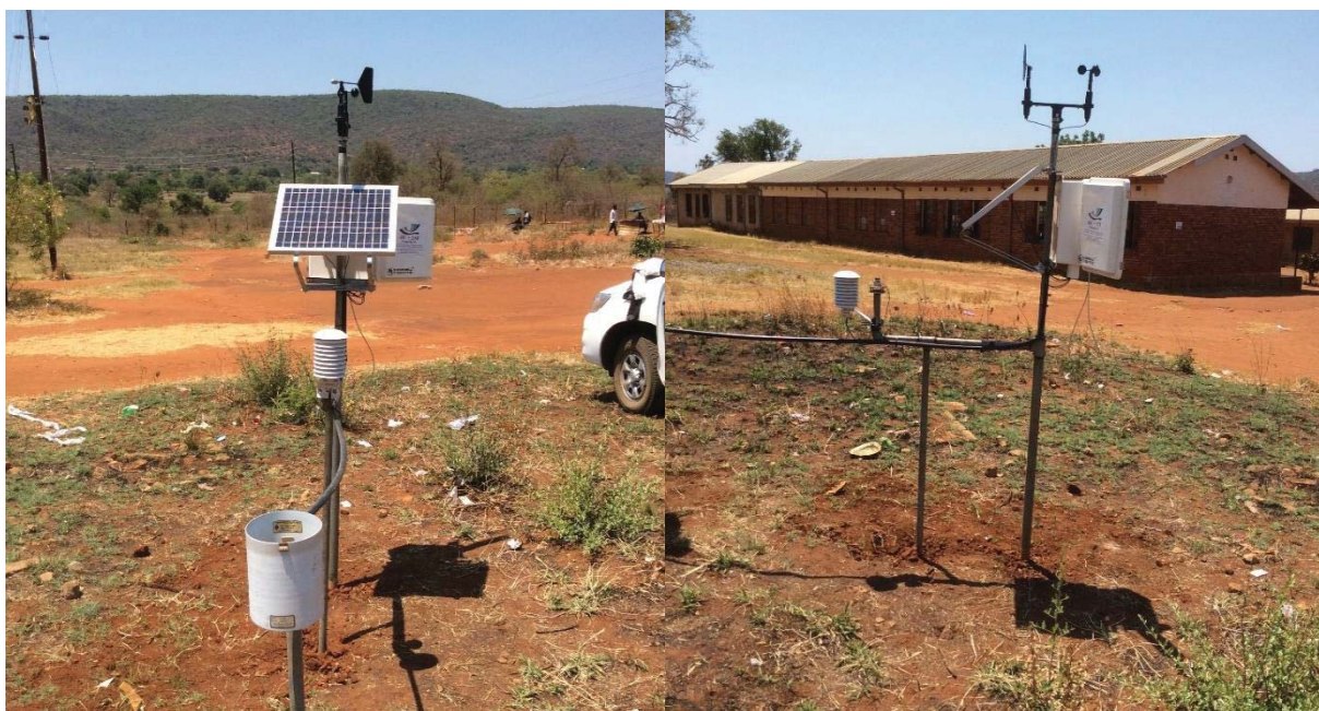
Figure 5: Installed weather station at Sumbana Secondary School (Lamvi)
