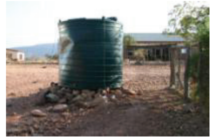
Figure 2.4c: Communal water storage tank
