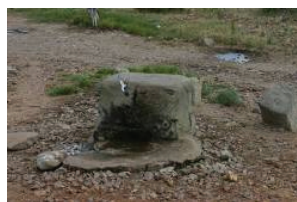
Figure 3.4c: Communal tap strengthened
