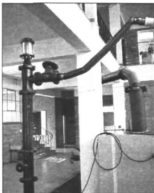
Figure 4.2.12: The extended supply pipe and improved angle of lay-flat hose
