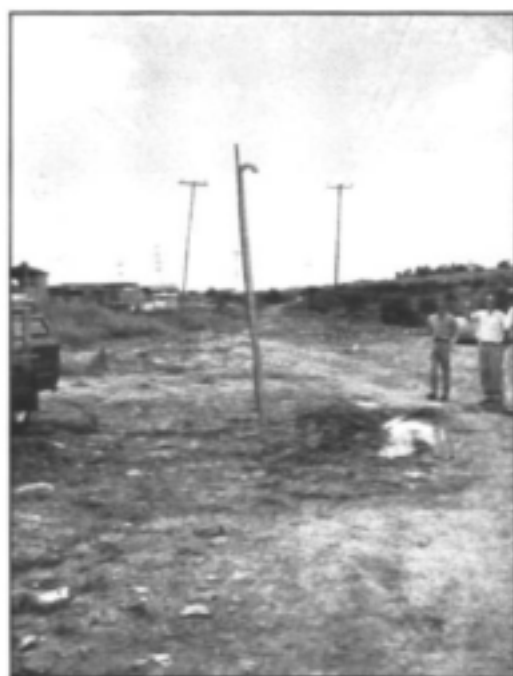
Figure 3.4.5: Standpipe with indication of spillage
