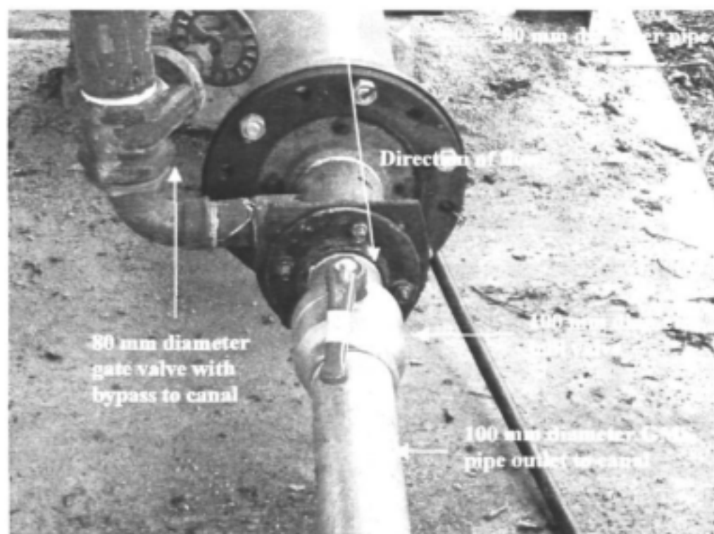
Figure 4.4.4: Ball valve to create the negative surge wave
