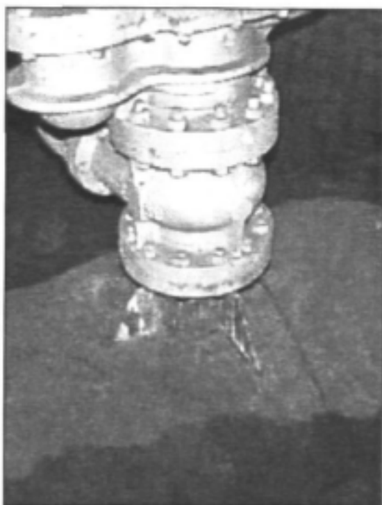
Figure 3.3.4: Typical combination air valve
