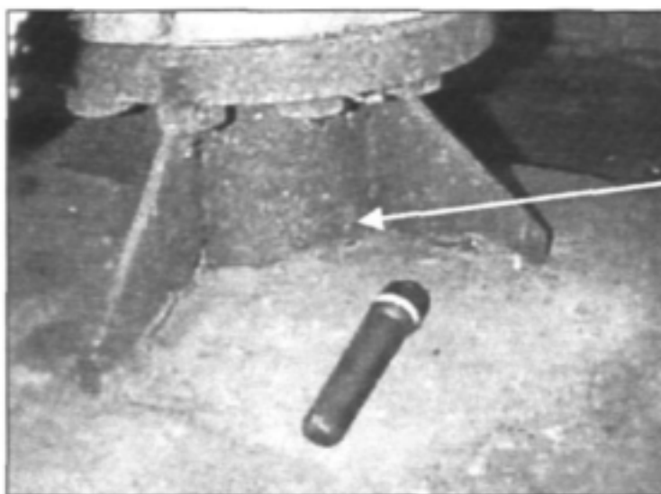
Figure 3.3.2: Typical 200 mm off take (stub) underneath the air valve
