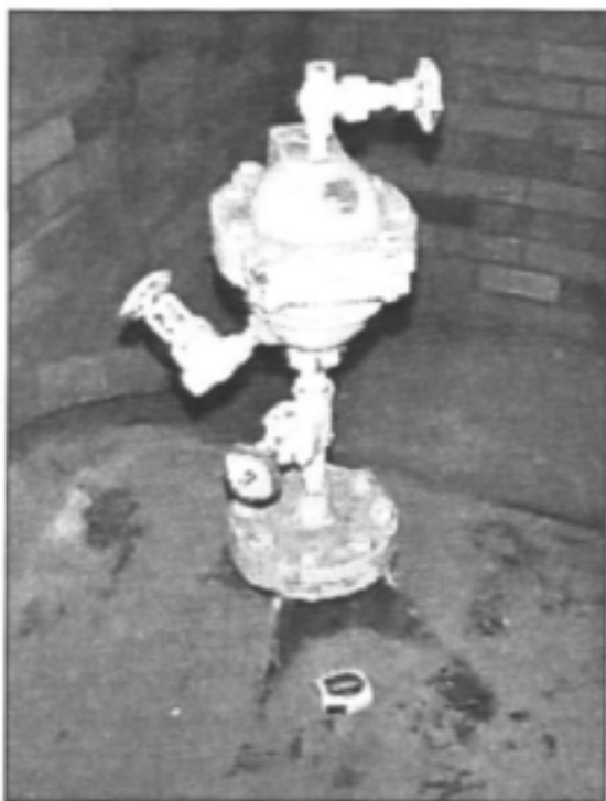
Figure 3.3.3: Typical small orifice air valve
