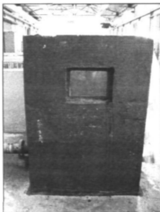
Figure 4.3.4: Detail C of the schematic drawing (Figure 4.3.1) showing the transparent air valve installed on the off-take
